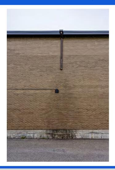
Protect masonry near gymnasium from further water damage by replacing missing brick and installing roof leaders with heavy duty downspouts designed to handle runoff and redirect water from sidewalk (preventing hazardous surfaces).
