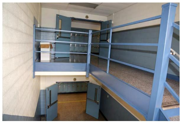
Install properly spaced stairway guardrails to comply with safety code and be ADA compliant.
