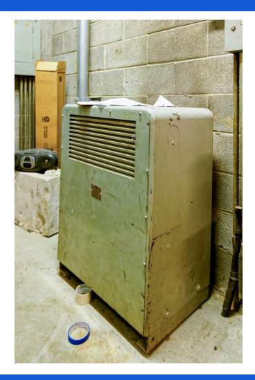
Replace end-of-life transformers (including a circa 1958 step-up transformer) and electrical panels to prevent power failure.
