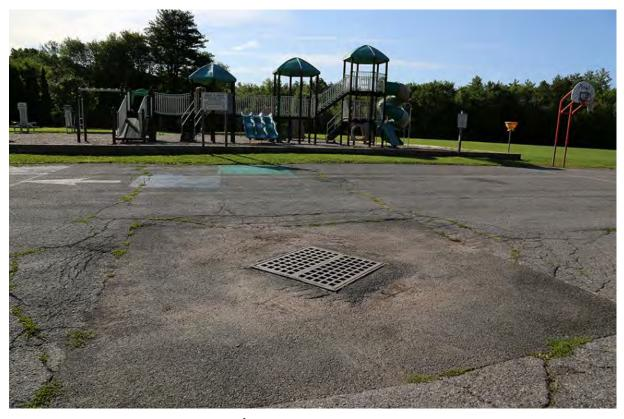
Resurface playground/student drop-off area (circa 1962) to remediate cracked and heaving asphalt and eliminate tripping hazards.
