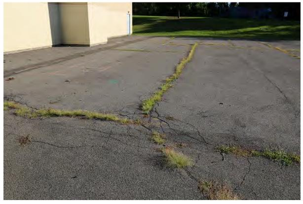
Resurface playground area to correct cracked and heaving asphalt to eliminate tripping hazards. Asphalt is original to the building and has exceeded its useful life.
