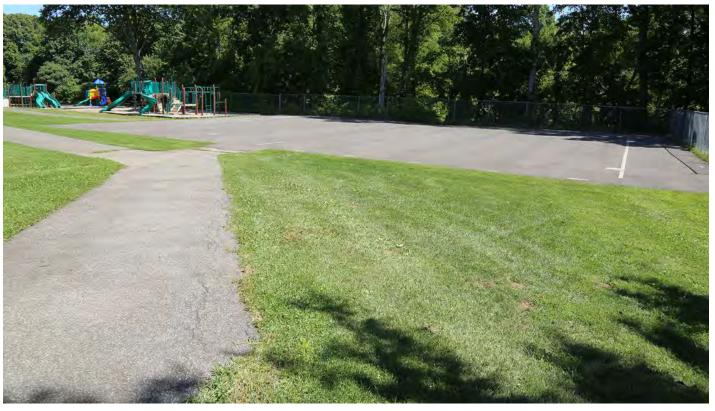
Resurface playground area to correct cracked and heaving asphalt and eliminate tripping hazards.
