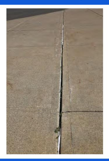
Protect the front sidewalk from deterioration caused by water infiltration by caulking existing joints.
