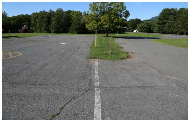
Replace aged and deteriorated pavement at the South Entrance, including providing drainage improvements to prevent further deterioration.
