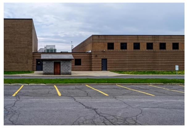
Remove existing deteriorating asphalt in the South Parking Lot and repave/restripe, including realigning a portion of the entrance drive to align with the Hildebrandt Building. Replace damaged concrete curbing and add concrete collars to all catch basins. Upgrade to heavy-duty pavement in the back portion of entrance drive and address drainage issues to prevent further deterioration. Install curbing and ramps to comply with Americans with Disabilities Act (ADA) requirements.
