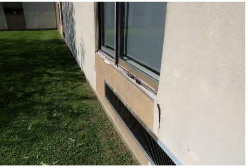
Reconstruct deteriorating exterior walls at the 100, 200, and 300 wings (remediate water infiltration) and replace rotting interior walls.
