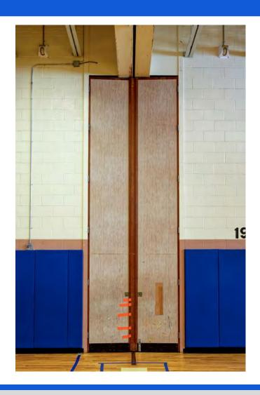
Remove original (circa 1965) manual folding gym partition and safety system and replace with an overhead curtain and new safety system. The existing partition does not operate properly and requires an expensive annual certification.
