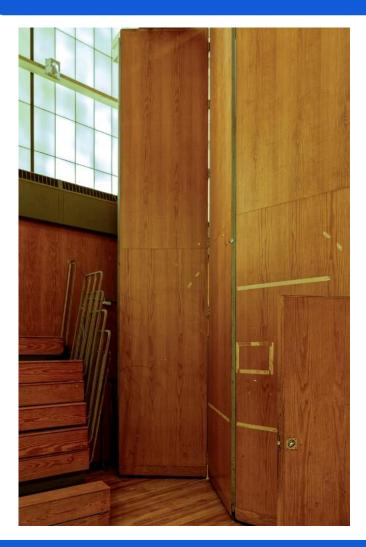
Upgrade non-functioning manual folding gym partition and safety system to provide an alternative solution (the existing partition does not operate properly and requires an expensive annual certification).
