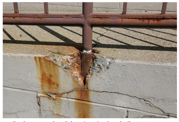
Replace rusted and deteriorating handrails at entrance ramp and back stairs, ensuring Americans with Disabilities Act (ADA) compliance.
