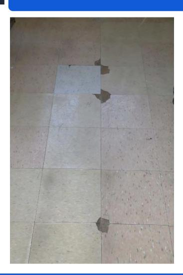
Replace cracked and deteriorating flooring, including plywood substrate.
