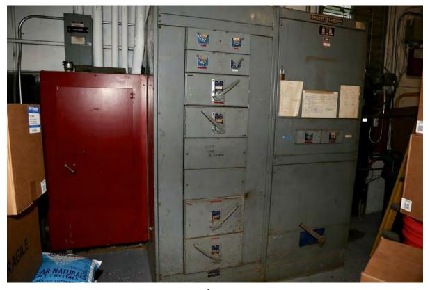
Upgrade the antiquated main distribution/circuit panel in the boiler room. This panel is original to the building and parts are obsolete. Reposition new panel to eliminate contact with water during frequent flooding. This is the last panel to be replaced in the District's buildings.
