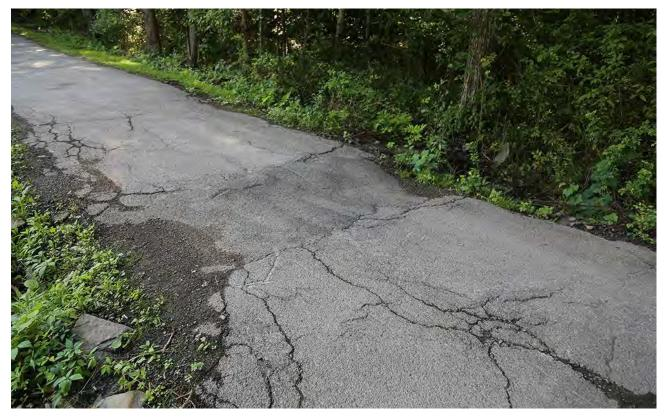
Reconstruct heaved and deteriorated asphalt walkway along Harry Wells Rd. toward Buffalo Rd., including the replacement of a collapsed culvert pipe that poses safety concerns.
