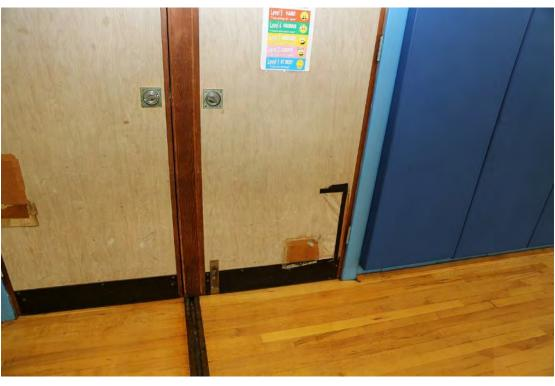
Replace an antiquated folding gym partition that is original to the building with an easily movable overhead curtain.
