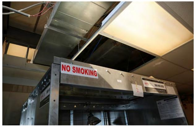
Provide ventilation ductwork for an existing paint booth in the Technology classroom, including abatement of the tar paper used on the roof and providing electrical connections.
