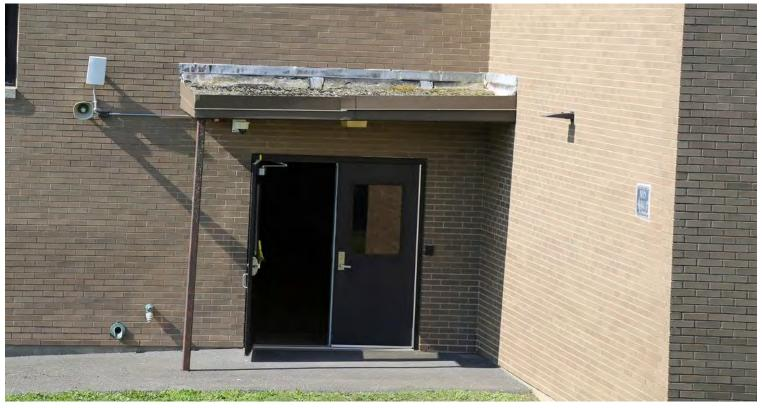
Replace identified canopy soffits (including roofing) to redirect water away from electrical components and reduce sidewalk hazards created by pooling water.
