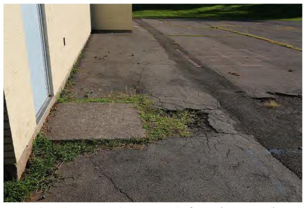
Replace deteriorated concrete platforms (circa 1965) by both gym exits.
