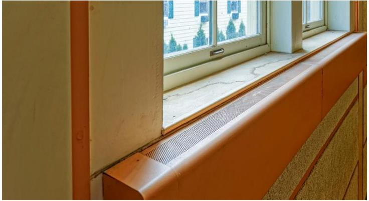
Expand heating capacity in perimeter rooms by adding additional finned tubes to radiation heaters. The current finned tubes are undersized for the rooms.
