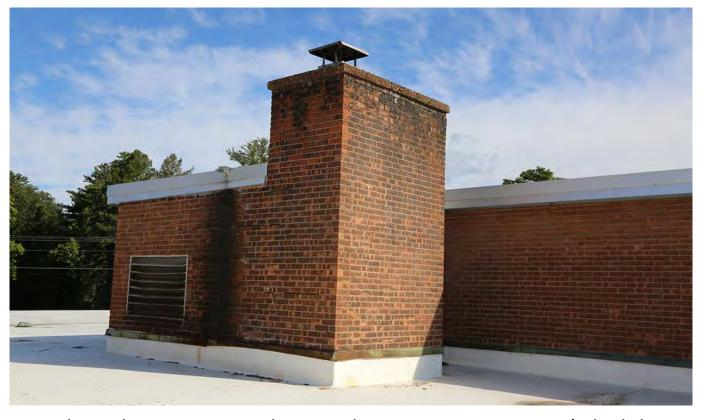
Replace chimney cap and repair deteriorating masonry (which has loose and spalling bricks), providing a seal from weather elements and protecting the building's integrity.
