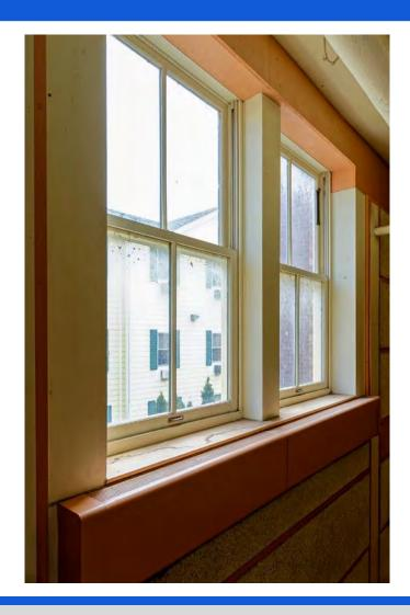
Upgrade rotting and thermally inefficient windows, many of which are wooden and non-functional.
