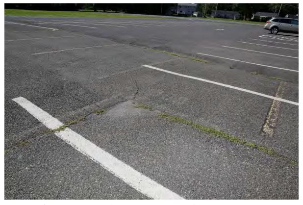
Grade, repave, and restripe East Parking Lot to correct deteriorating blacktop, which is over 25 years old and has reached its end of life.
