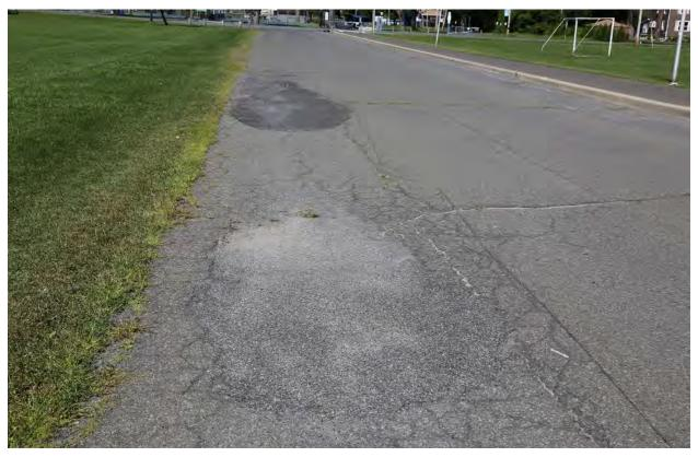
Remove existing heaving and cracking asphalt in the Bus Circle and repave/restripe; address drainage issues that are causing deterioration.
